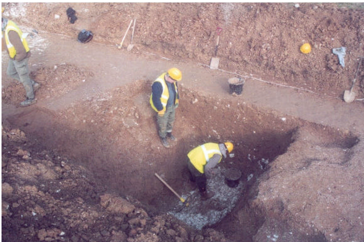
Figure 9. Area 1 Section 5 under excavation, from North
